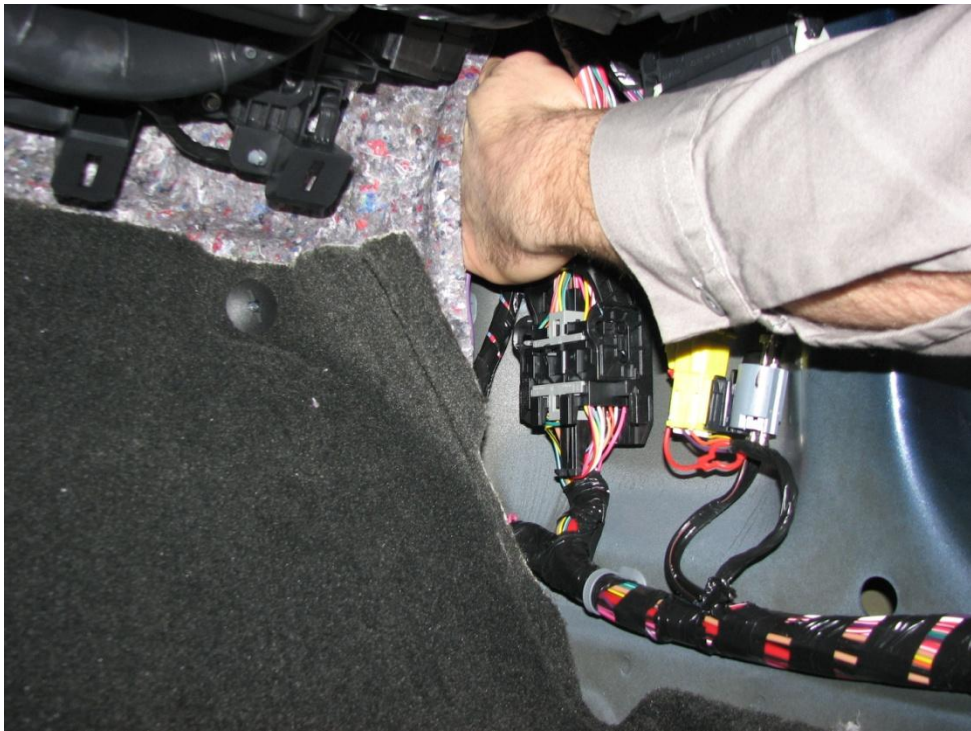
Photo 12: Reach hand behind insulation to feel for grommet
