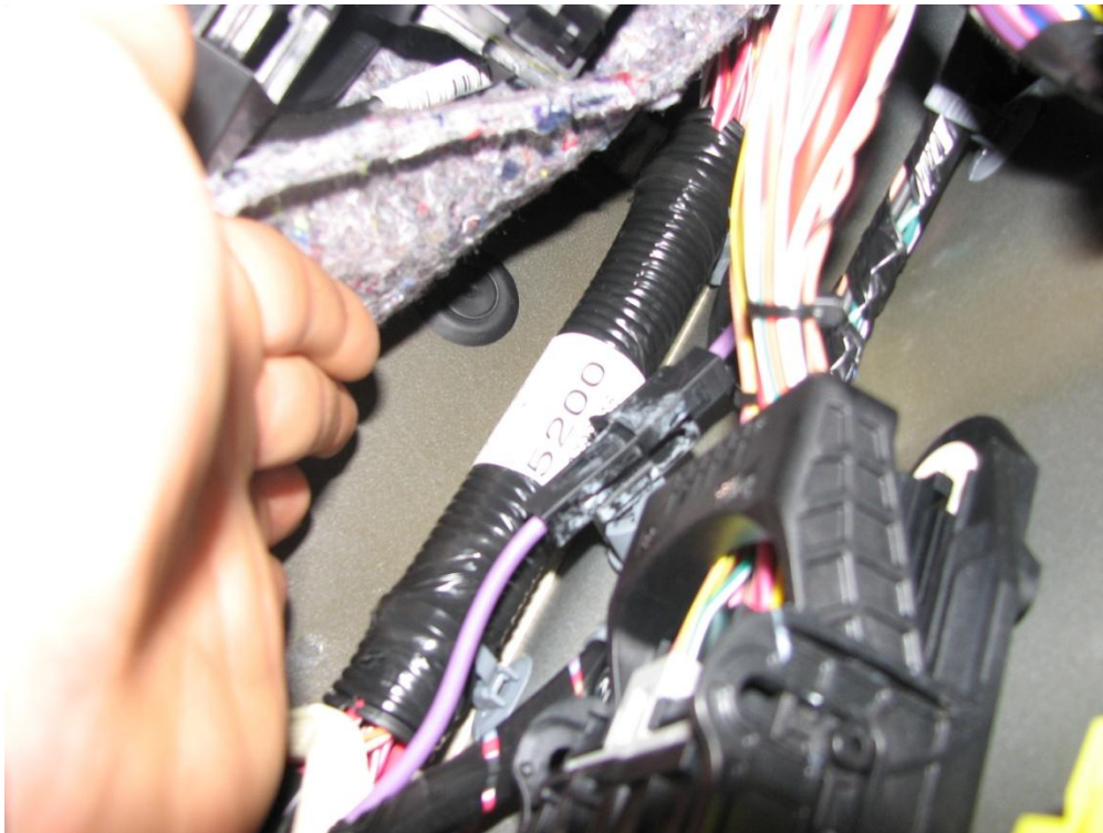
Photo 13: Grommet to be removed and drilled
