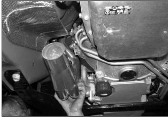
Figure 3: Insertion of driver's side header
