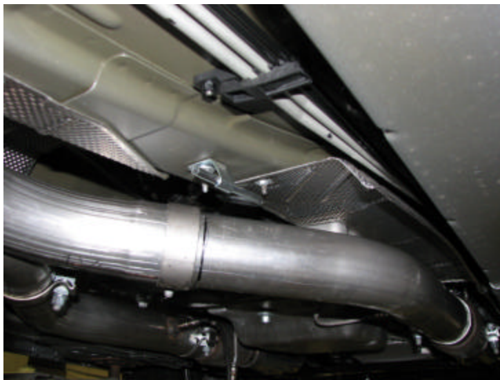
Figure 6: A/C drain line pushed up (shown after pipes have been installed)
