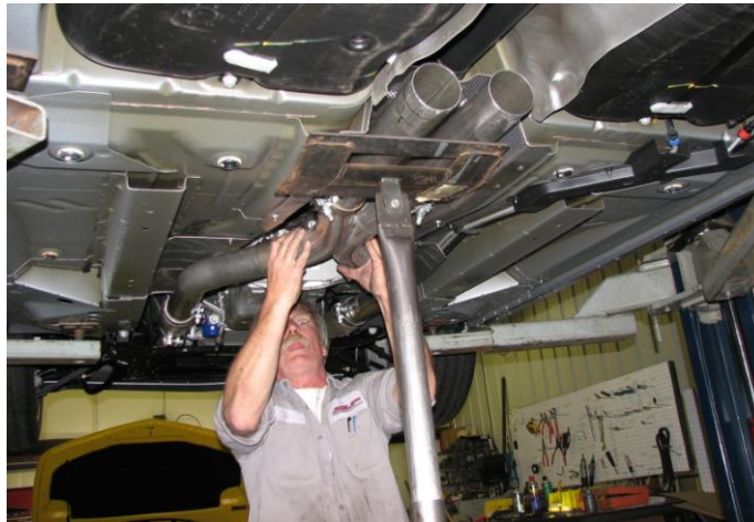
Figure 7: Installation of X-Pipe assembly
