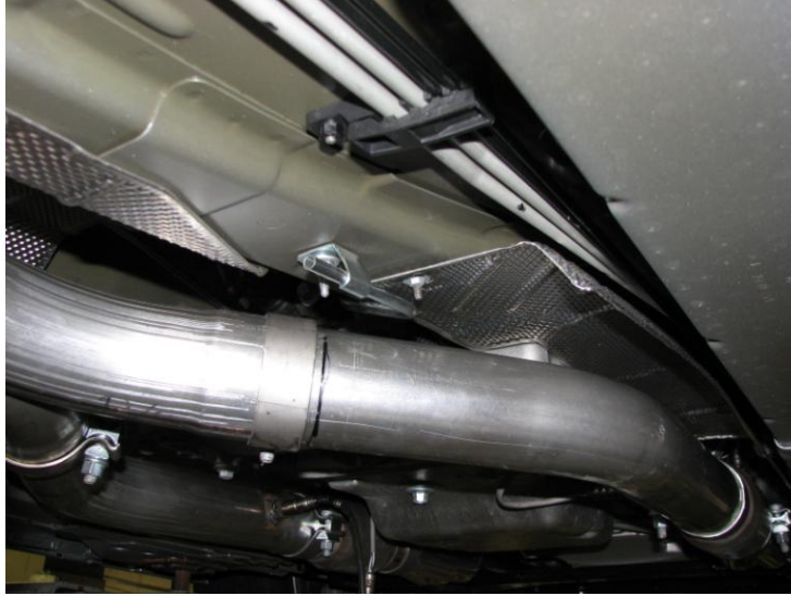
Figure 7: A/C drain line pushed up (shown after pipes have been installed)
