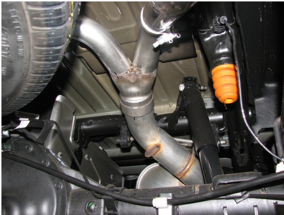
Figure 2: Installation of 'Y-pipe'
