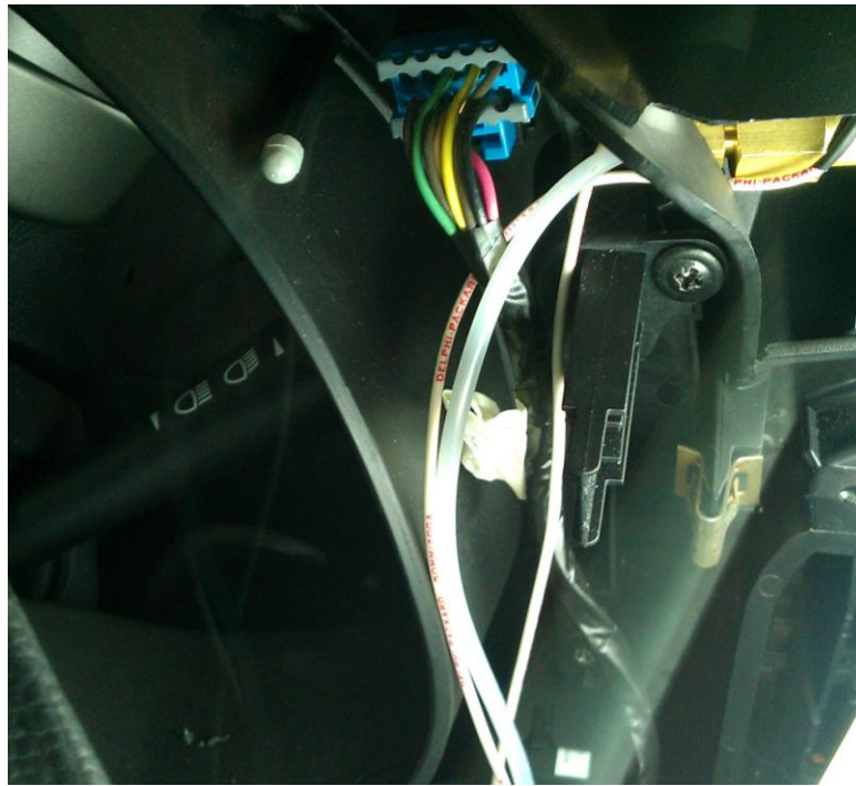
Figure 15: Power wires and vacuum line routing
