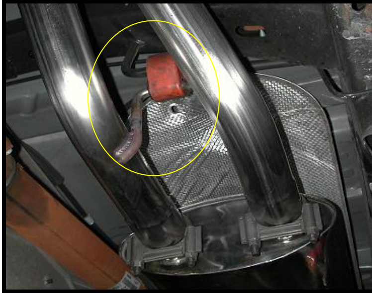
Photo 8: Over-axle Pipes Attached to Muffler
